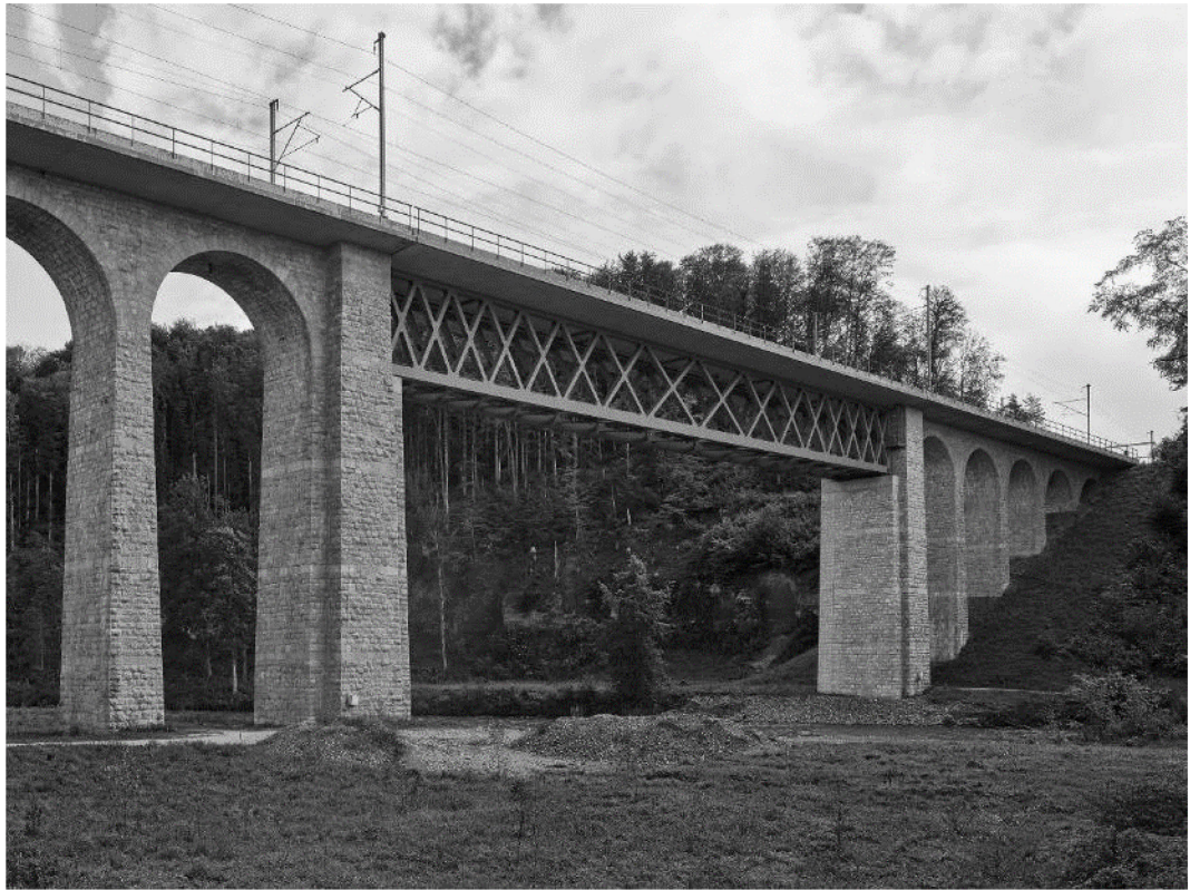
Fig. III.5 Saaneviadukt in Gümmenen, BE. © Ariel Huber Photography
